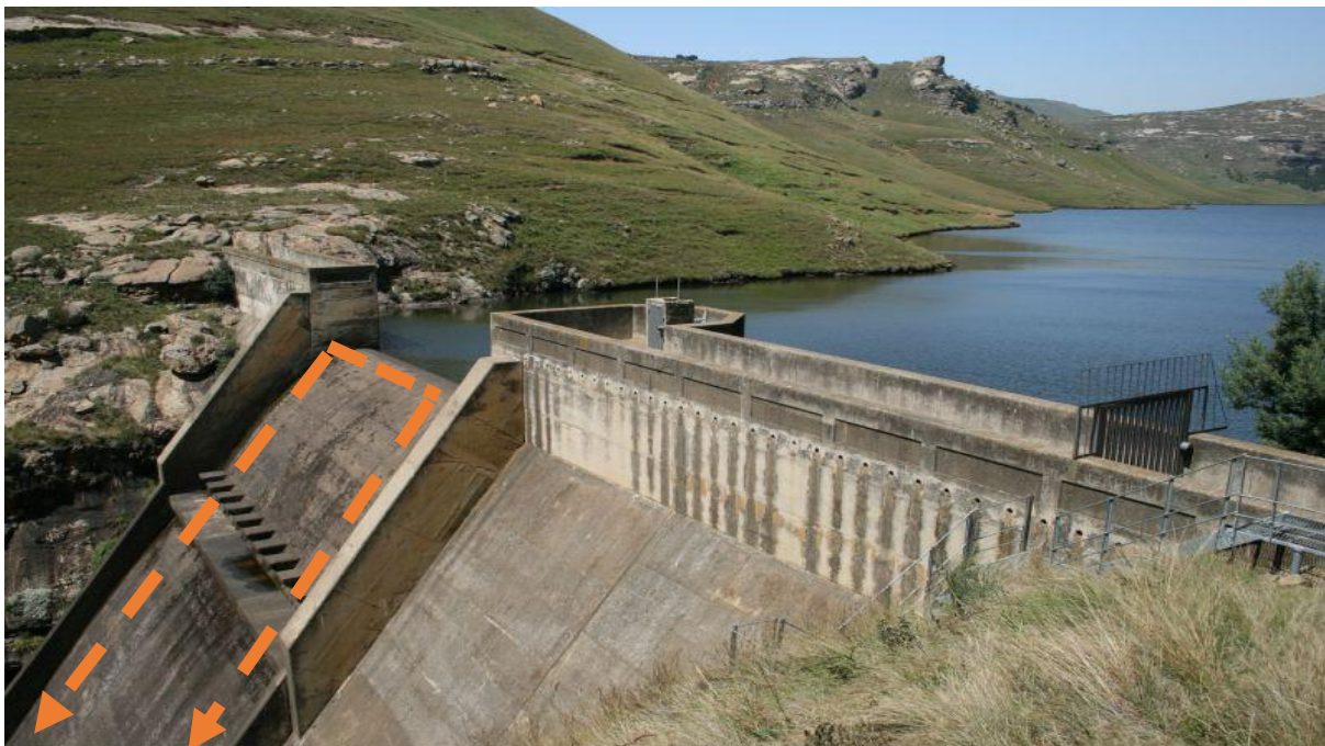
Figure 3: A spillway on the Metsi-Matsho Dam in the Free State Province
