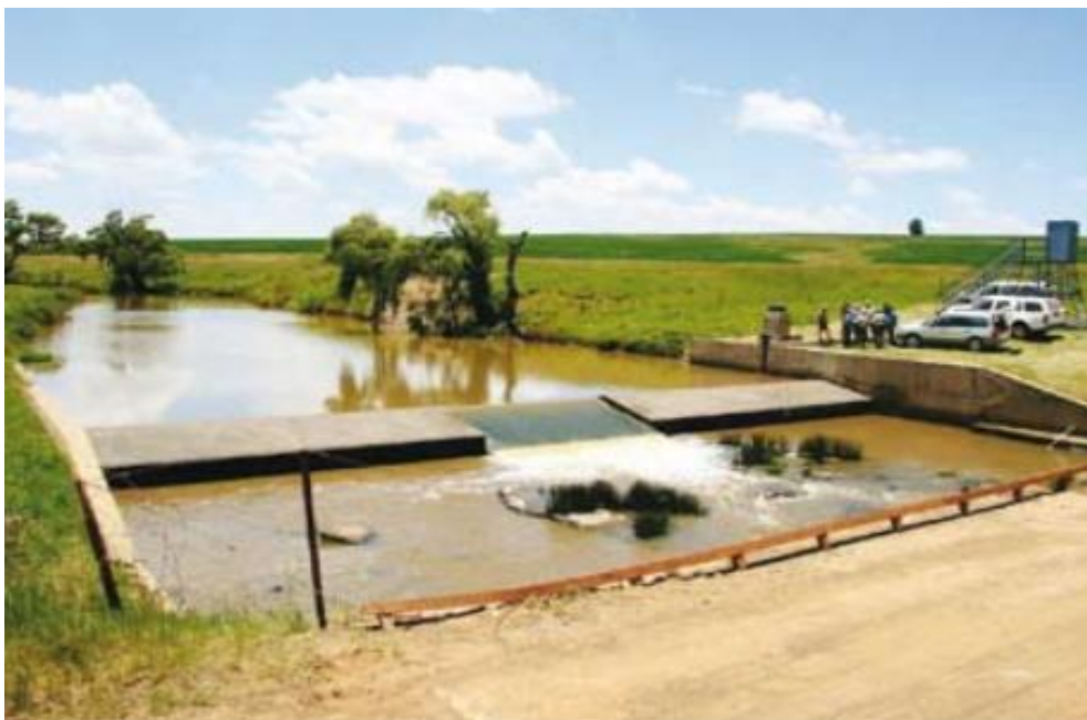
Figure 9: Example of a horizontal compound Crump weir without dividing walls in the Vaal River catchment (Mpumalanga)
