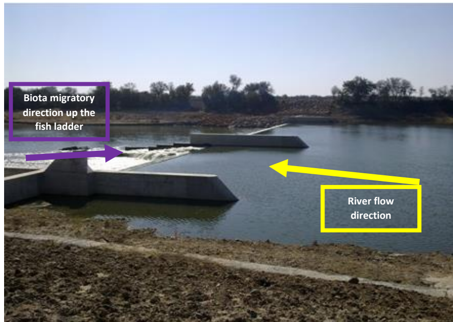
Figure 14: A typical example of a fish ladder Source: DWS Hydrological Services website, 2024
