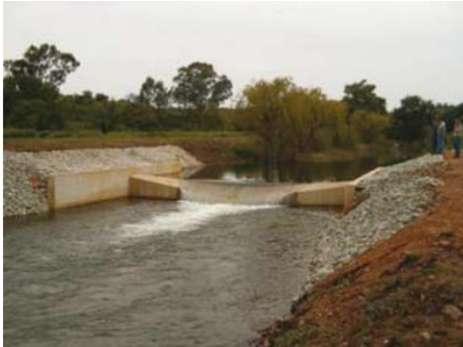
Figure 10: Example of a V-shape Crump weir in the Mooi River near Potchefstroom (North-West Province)
