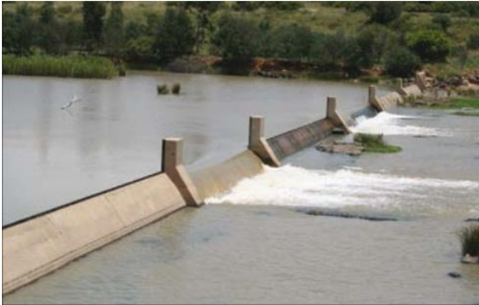
Figure 8: Example of a compound sharp-crested weir in the Vaal River downstream of Vaal Dam
